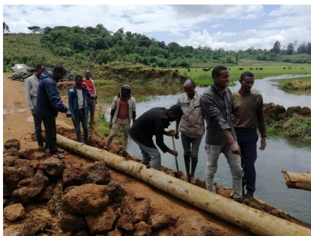
Figure 2 | Community members constructing a bridge for the drill rig
